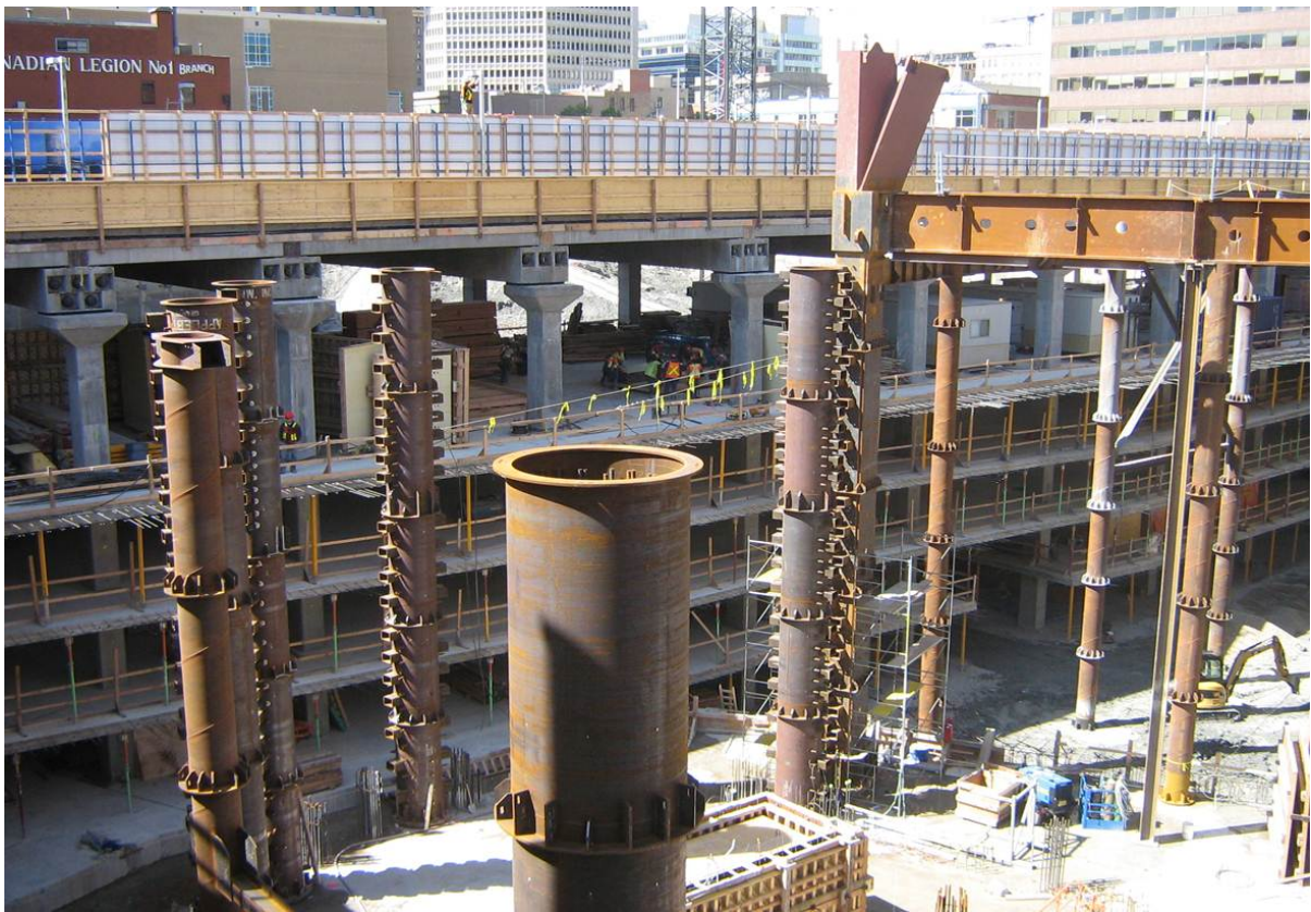
Top Down Construction (6 storey tall composite steel columns)
