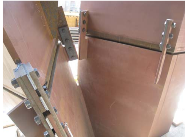
Various stages of the tower construction
