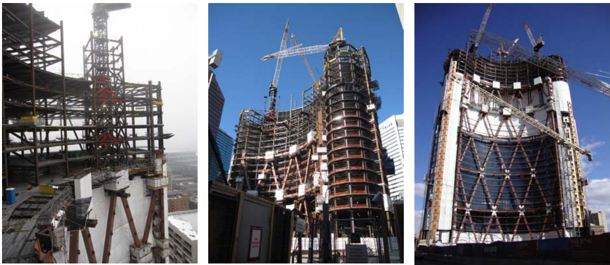
Various stages of the tower construction
