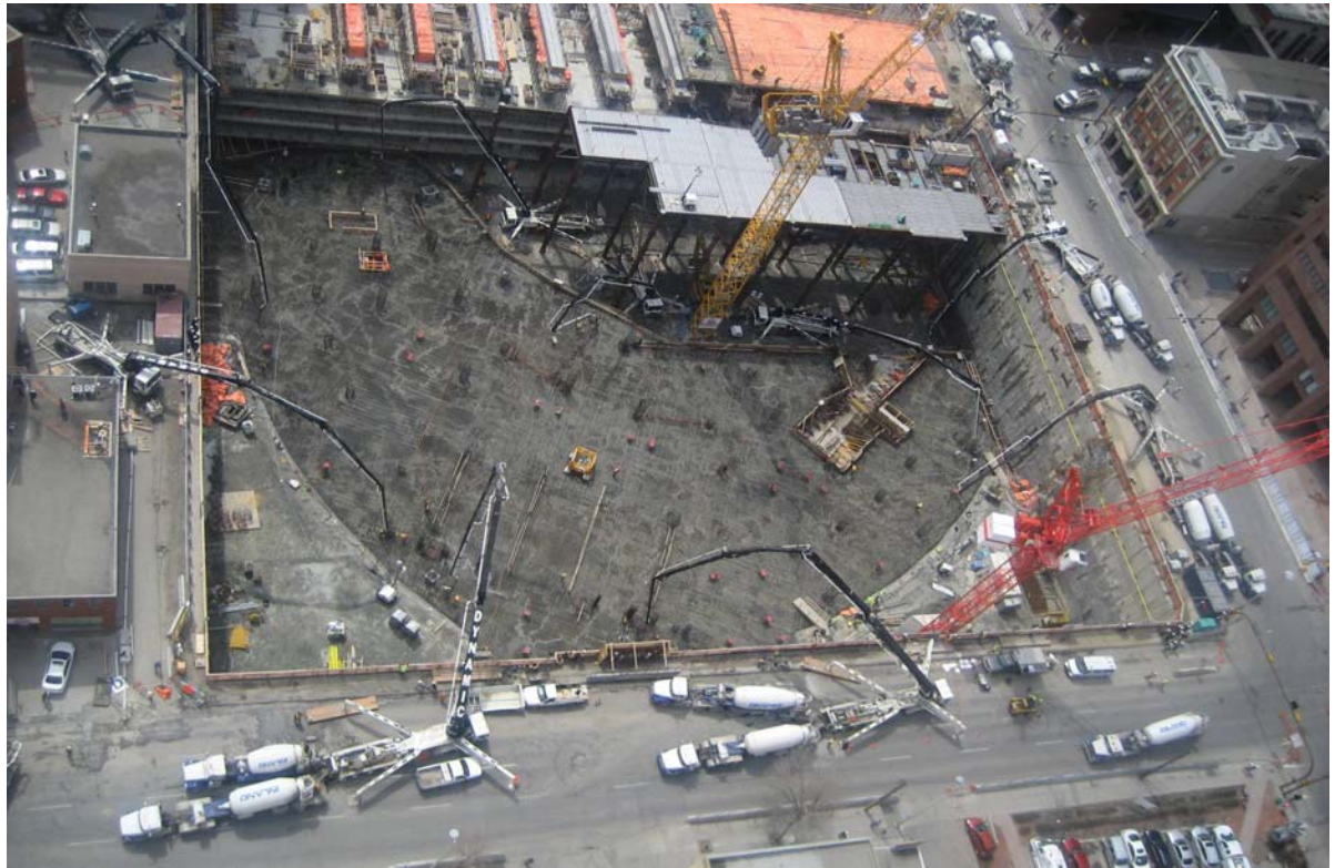
The Raft (a single pour, 40hrs, 14,000m 3 )
