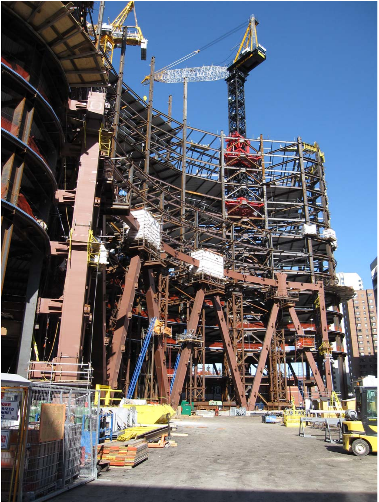
Structural Steel Construction Progress
