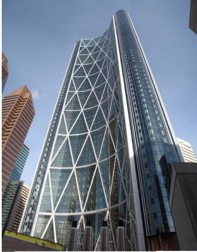
Expression of the diagonal elements of the atrium screen wall (Image provided by Foster + Partners)
