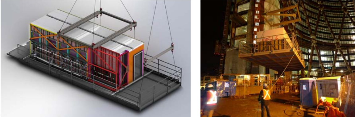
BIM image and on site hoisting of the modular washroom
